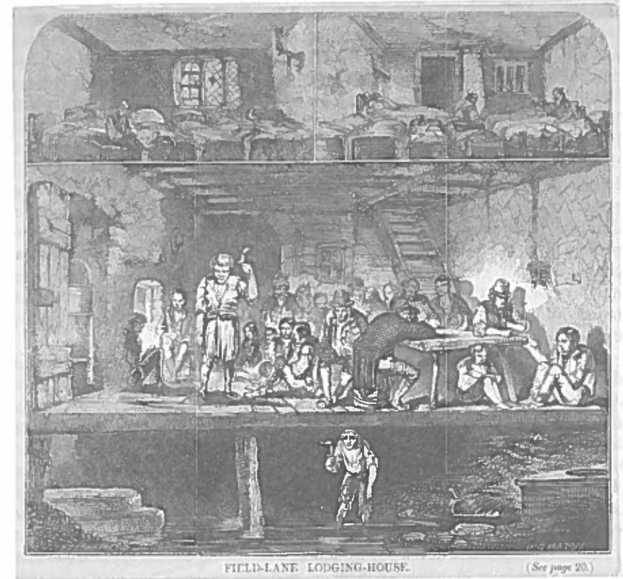
Figure 2.2 Open sewer running under lodging house in Field Lane, London. Reprinted with permission of the Guildhall Library, Corporation of London
